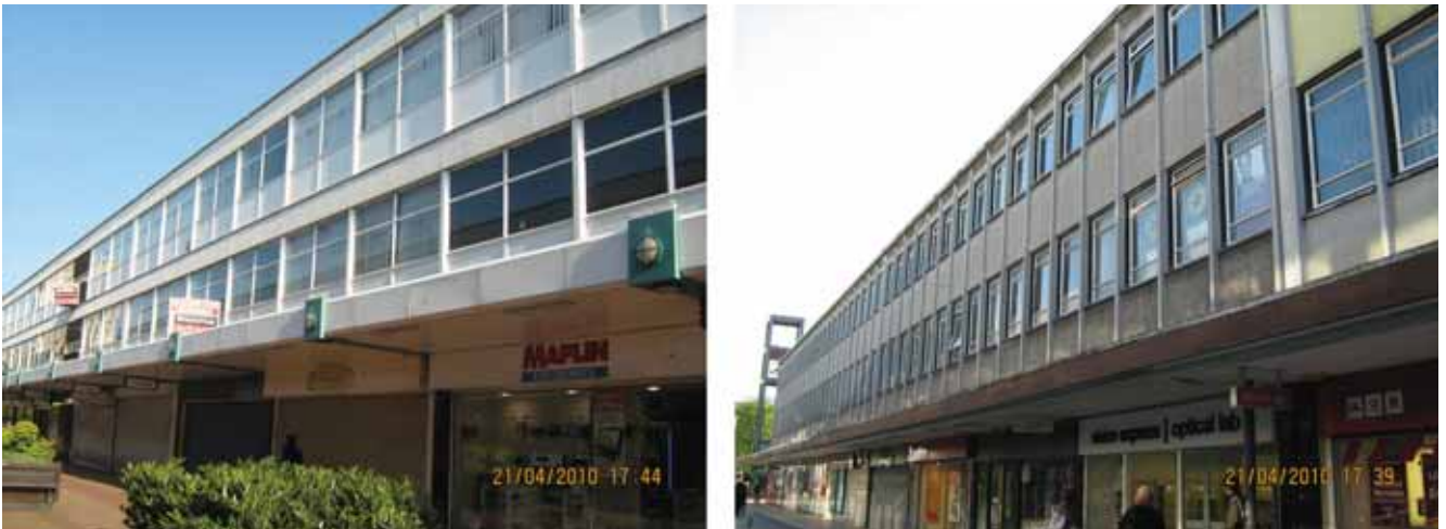
Typical building styles
