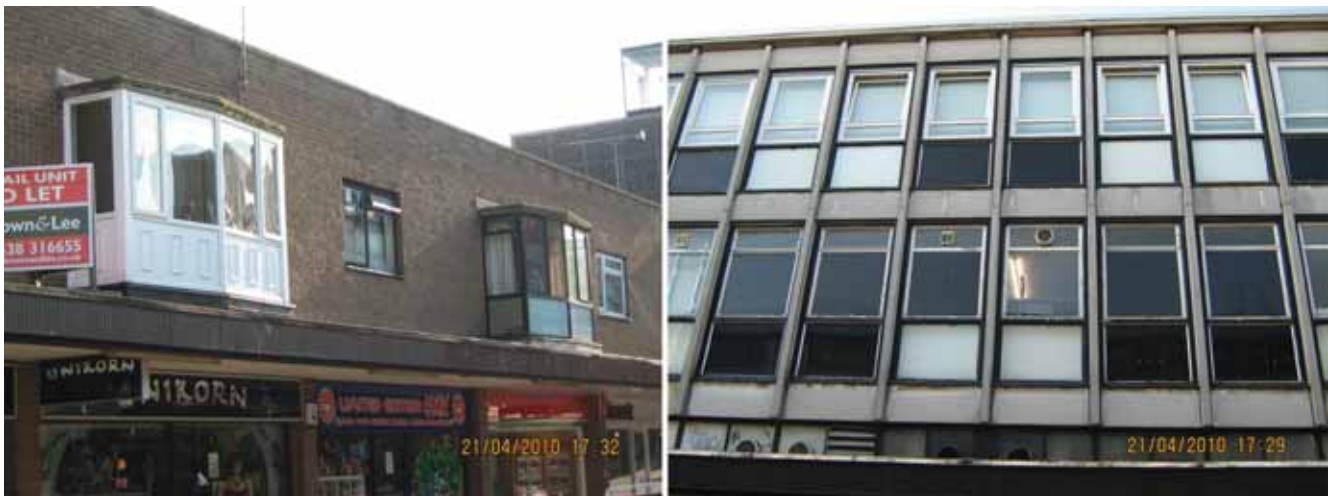
UPVC window installments set against original windows
