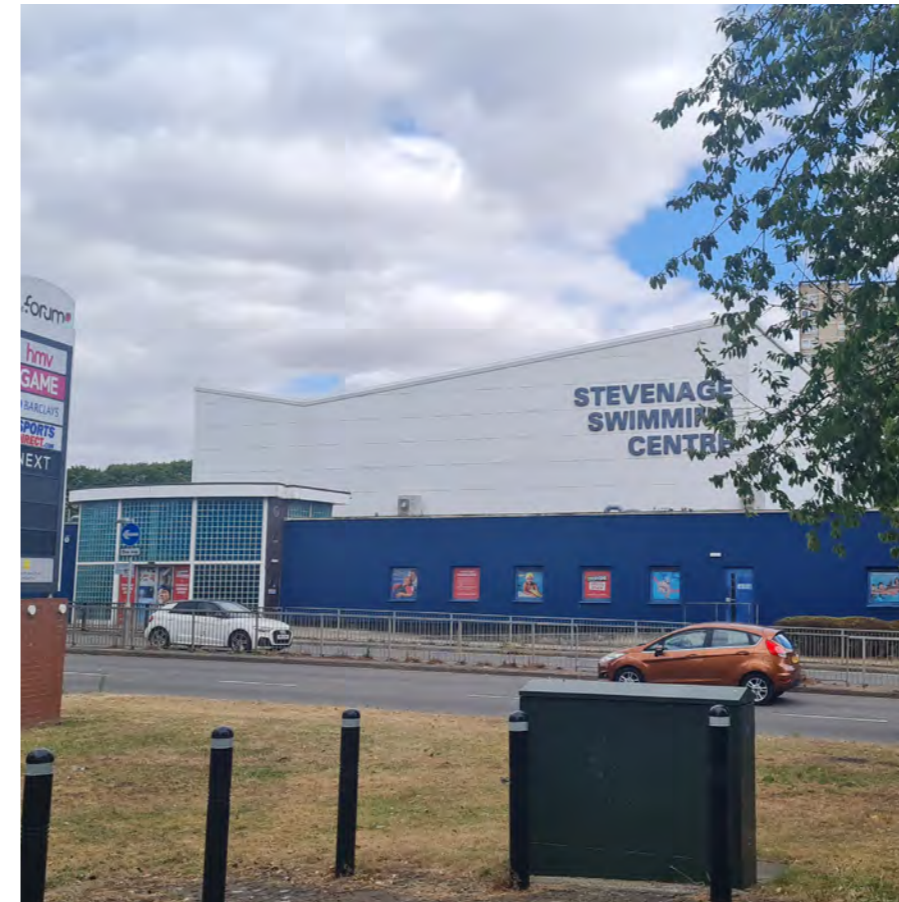
Existing Stevenage Swim Centre
