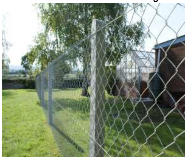
Picture 1 - Chain Link Fencing
