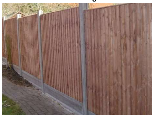
Picture 2 - 1.8m Panel Fencing with Concrete Post
